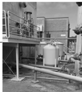
Siloxane treatment system (yellow vessels)
